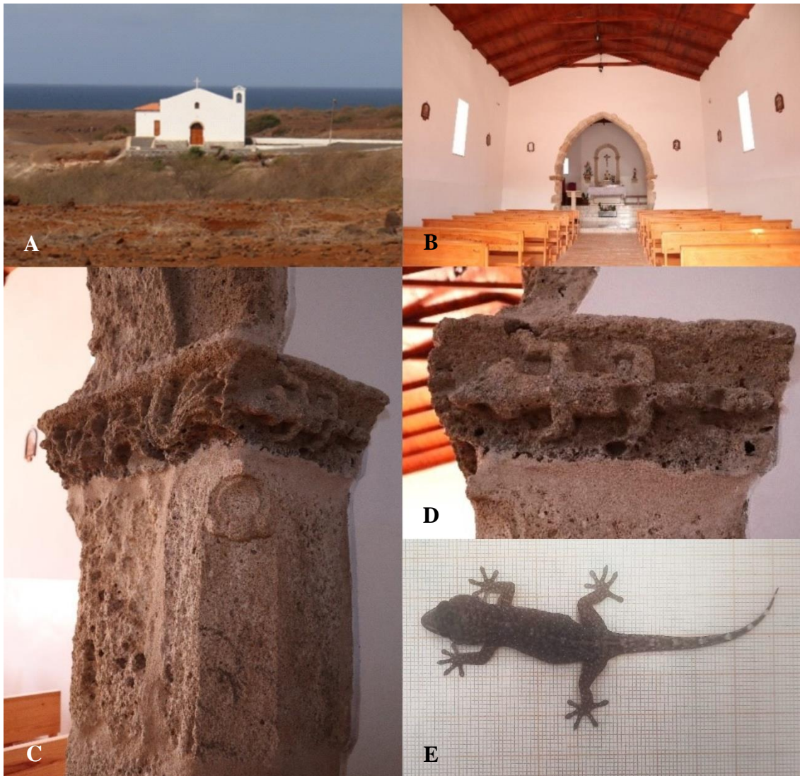
Fig. 1. Pictures of the church of Nossa Senhora da Luz and details of its architectural and biotic elements (photos by M. Pacheco). A) Surroundings of the church in Alcatrazes Bay, southeast of Santiago Island. B) Unhewn limestone pointed arch in the transition of the nave to the chancel with square, recessed columns with biotic representations in the chapters. C) The northern chapter with Acanthus leaves, a shell on the edge, and D) a gecko facing the altar. D) Photo of an individual of an endemic Tarentola species of Santiago.
